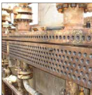
FinFan cooler before a maintenance
